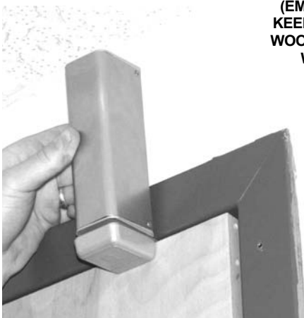
INSWINGING VERTICAL INSTALLATION. DEADBOLT ON FRAME FLUSH KEEPER ATTACHED TO TOP EDGE OF DOOR
