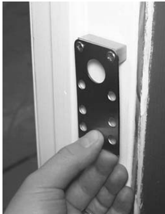
MORTISE KEEPER. MAGNET IS MORTISED (EMBEDDED) INSIDE THE DOOR FRAME AND KEEPER IS INSTALLED FLUSH. FOR USE WITH WOOD DOOR FRAMES ONLY. (METAL FRAMES WILL DISSIPATE MAGNET STRENGTH).
